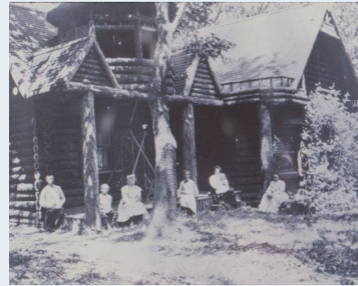
Full rehabilitation would bring the cabin back to as close to its original condition as possible
