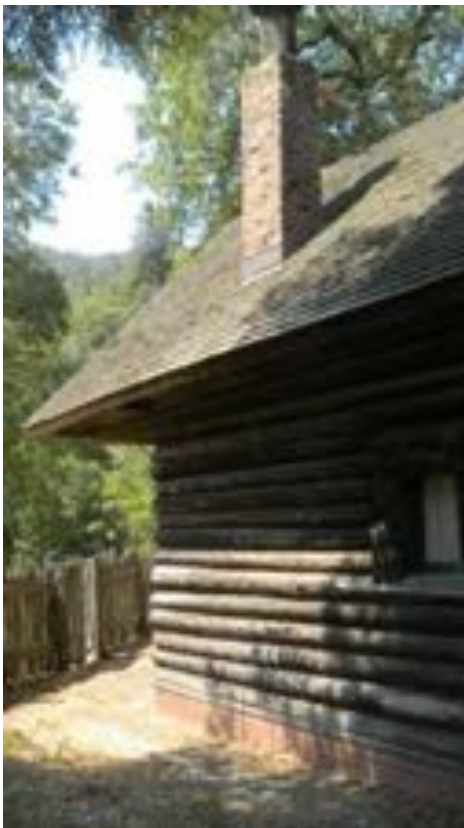
Fig.10 – PHOENIX CABIN - East side
