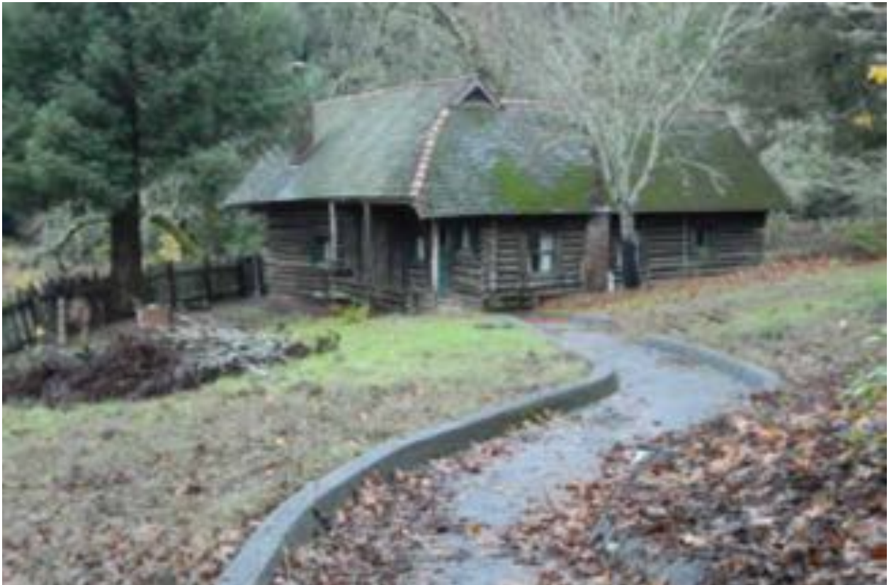
Fig.5 – PHOENIX CABIN - East side (left) and north/rear (right) from entry path, looking southwest
