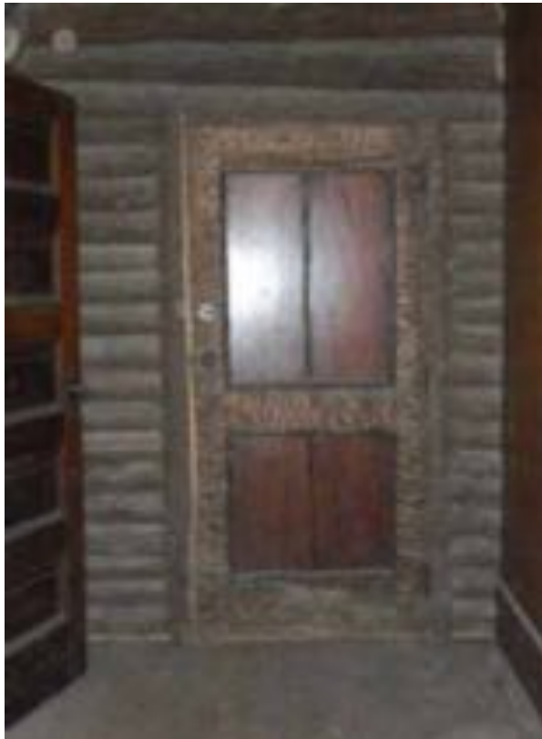
Fig.46 – Entry vestibule and door
