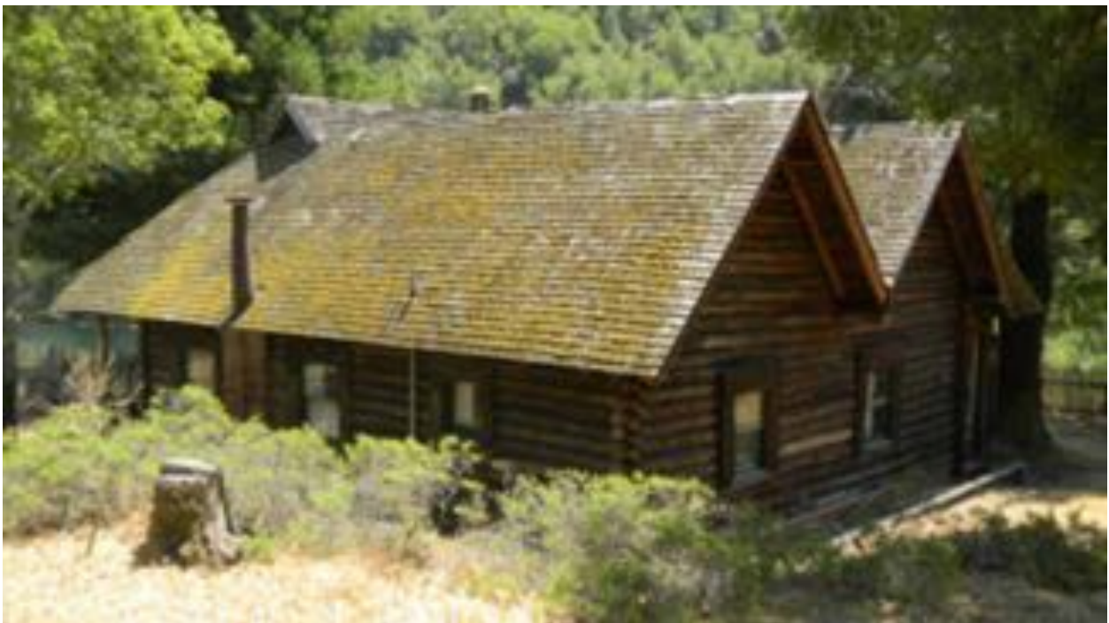
Fig.7 – PHOENIX CABIN - Rear/north (left) and west side (right), looking southeast
