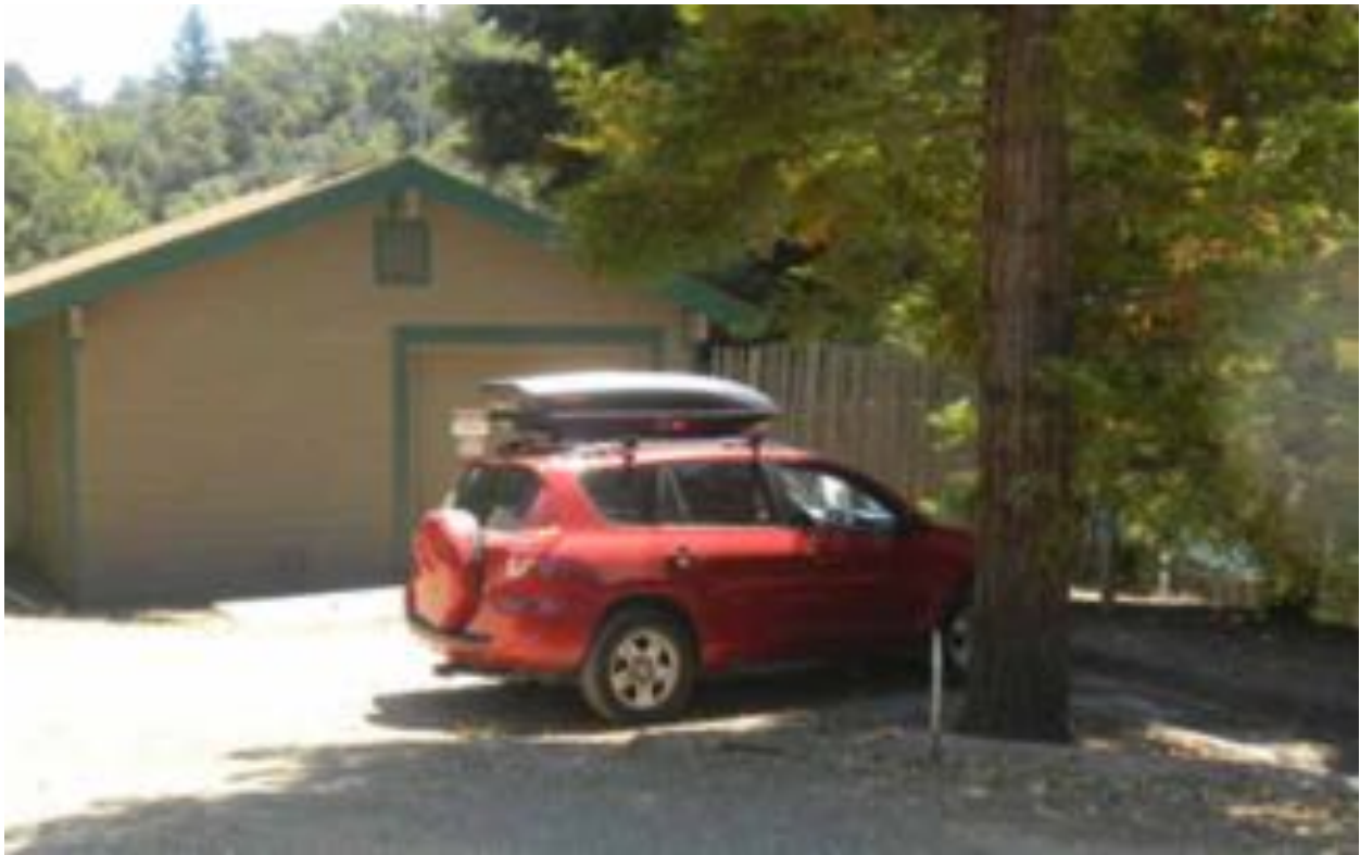
Fig.31 – Site - Accessible parking space above Cabin (pump house at left)
