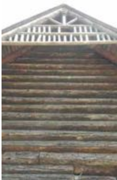
Fig.12 – Log work at front gable
