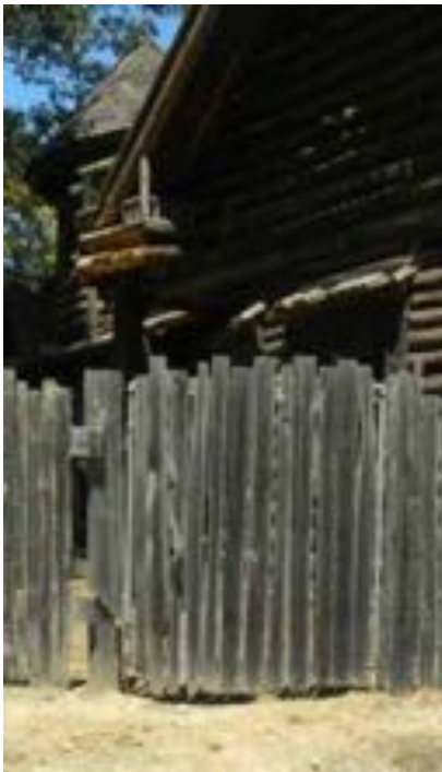
Fig.32 – Front gate & fence
