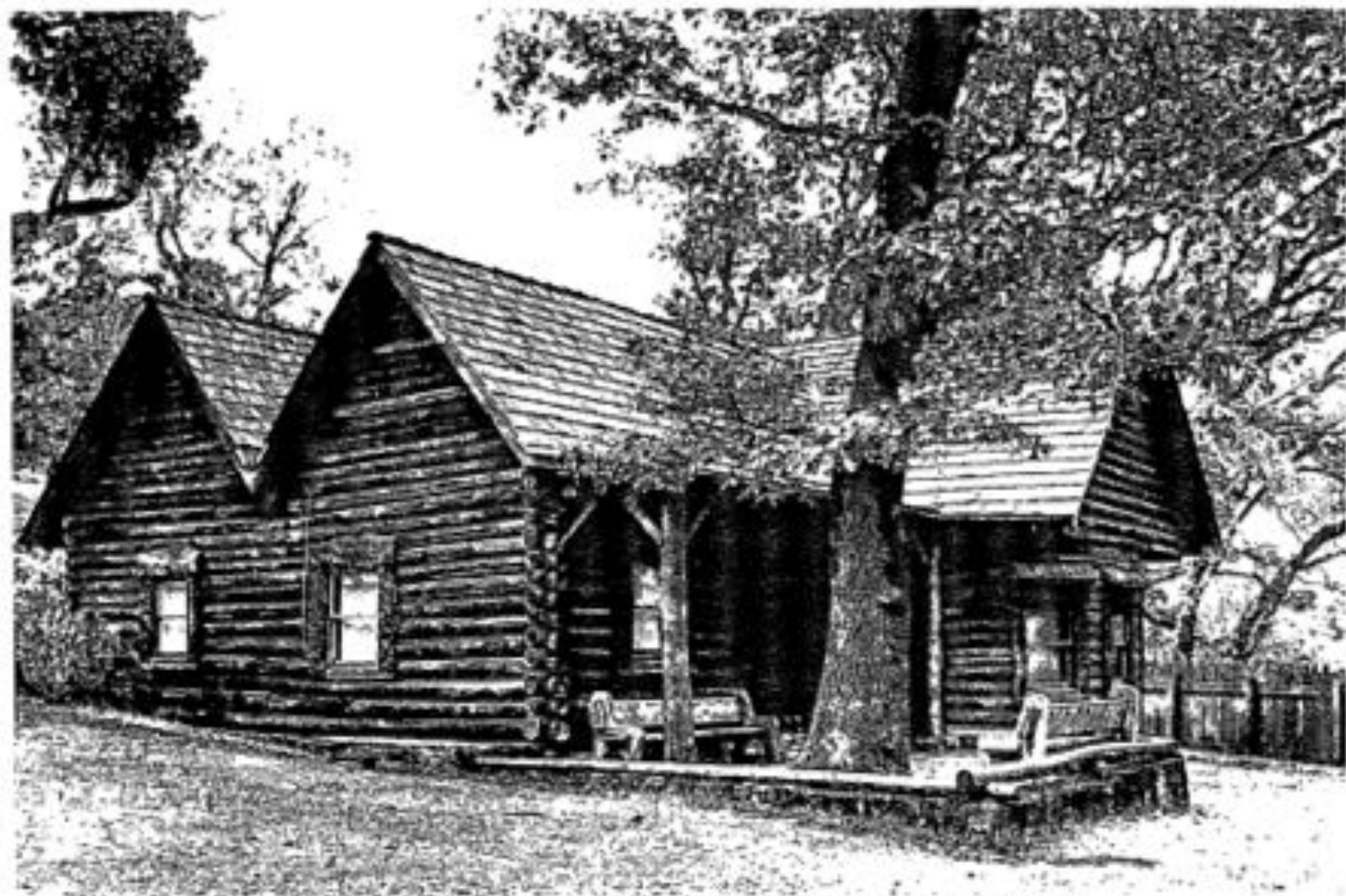
Southwest and northwest elevations looking east. Terrace is not original and the original wood porch (as seen in the c.1900 photograph) should be replaced.
