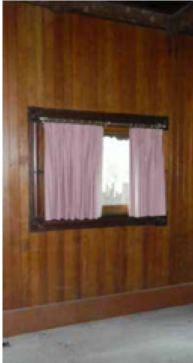
Fig.48 – Living room wall-window
