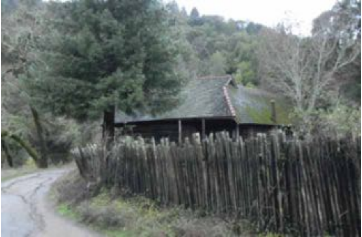
Fig.4 – PHOENIX CABIN - Northeast corner from fire road, looking southwest
