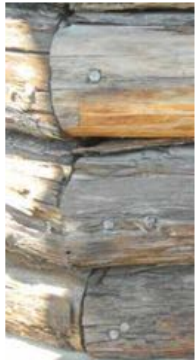
Fig.14 – Log work detail
