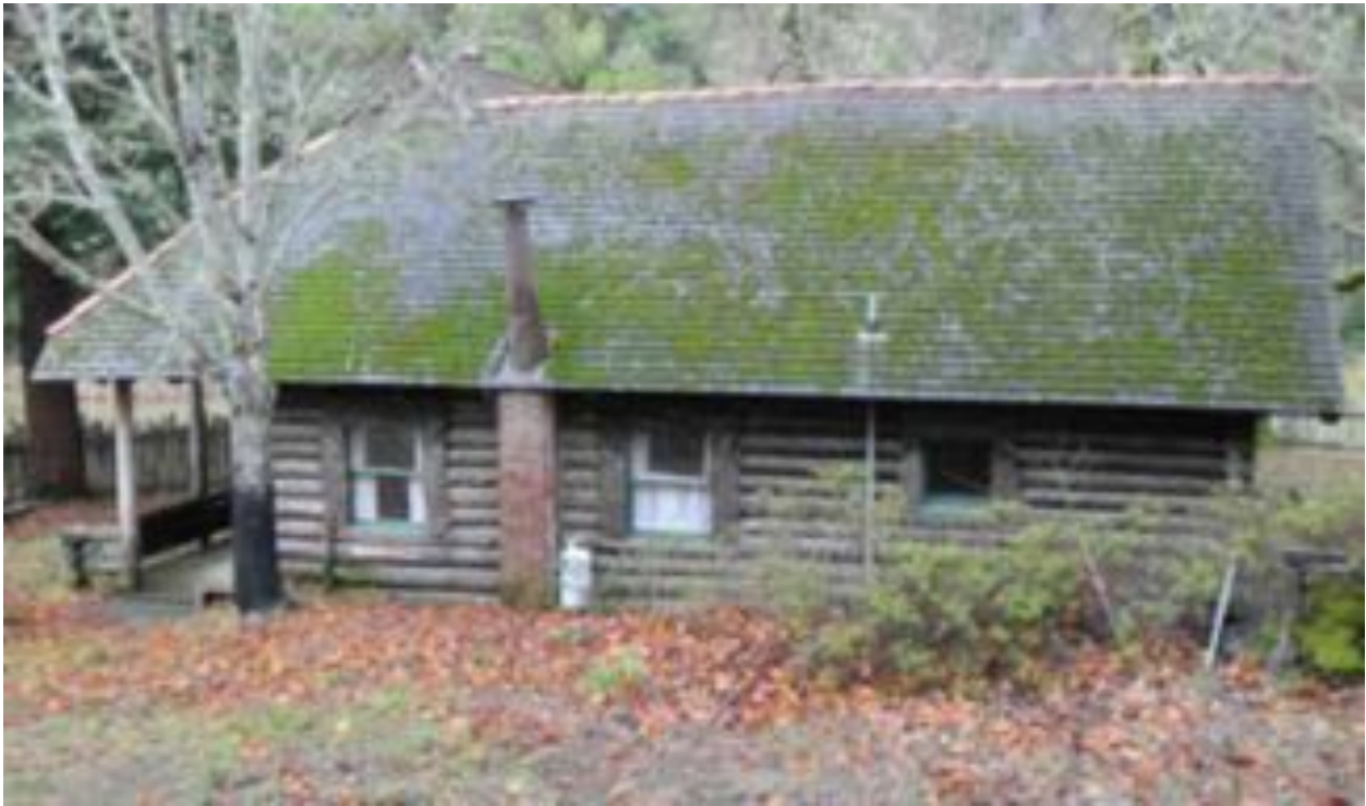
Fig.6 – PHOENIX CABIN - Rear/north, looking south
