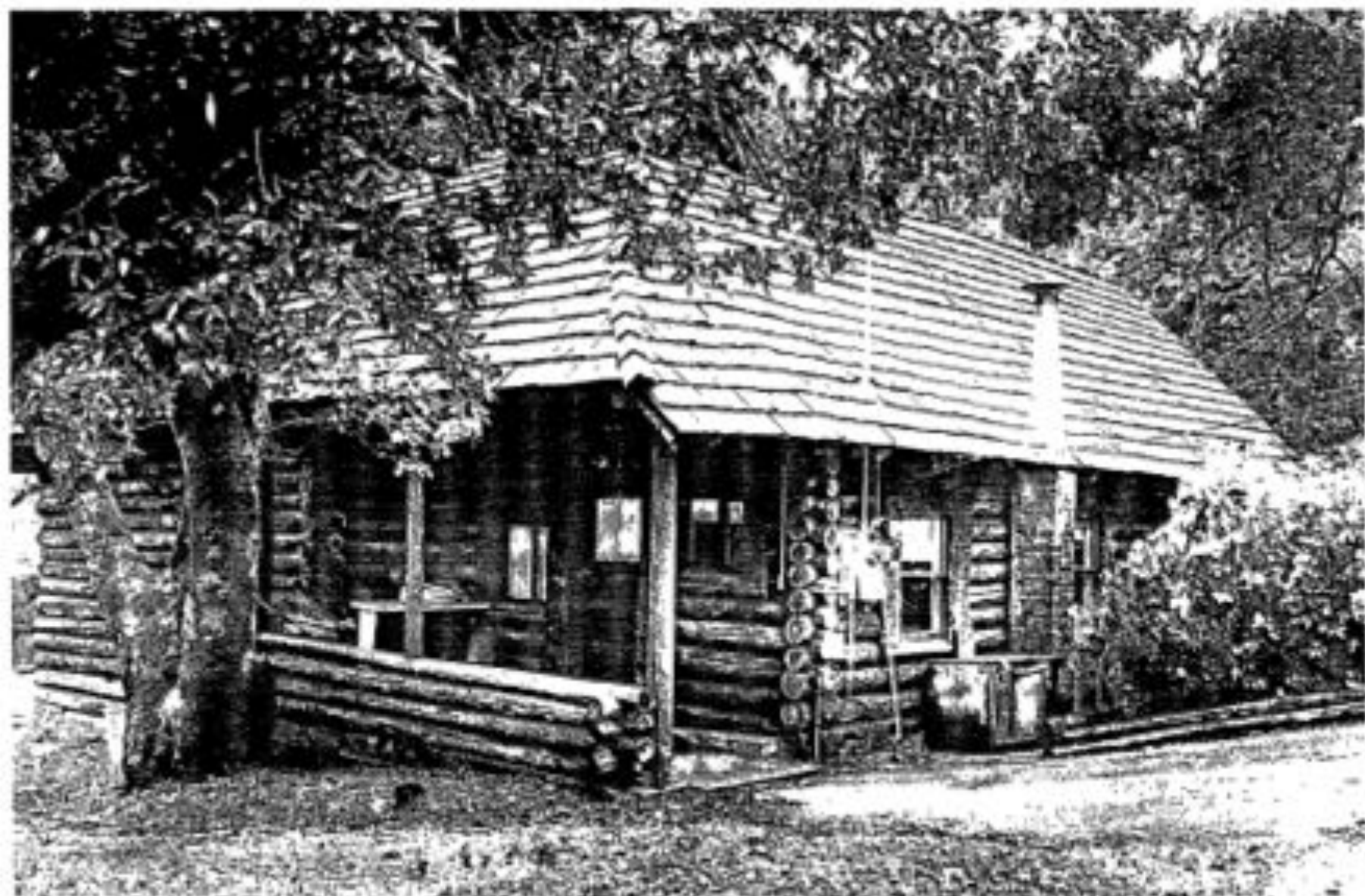
Northeast (rear) and southeast elevations looking west. Note unsightly electrical equipment and conduits--these should be relocated in a less conspicuous location.
