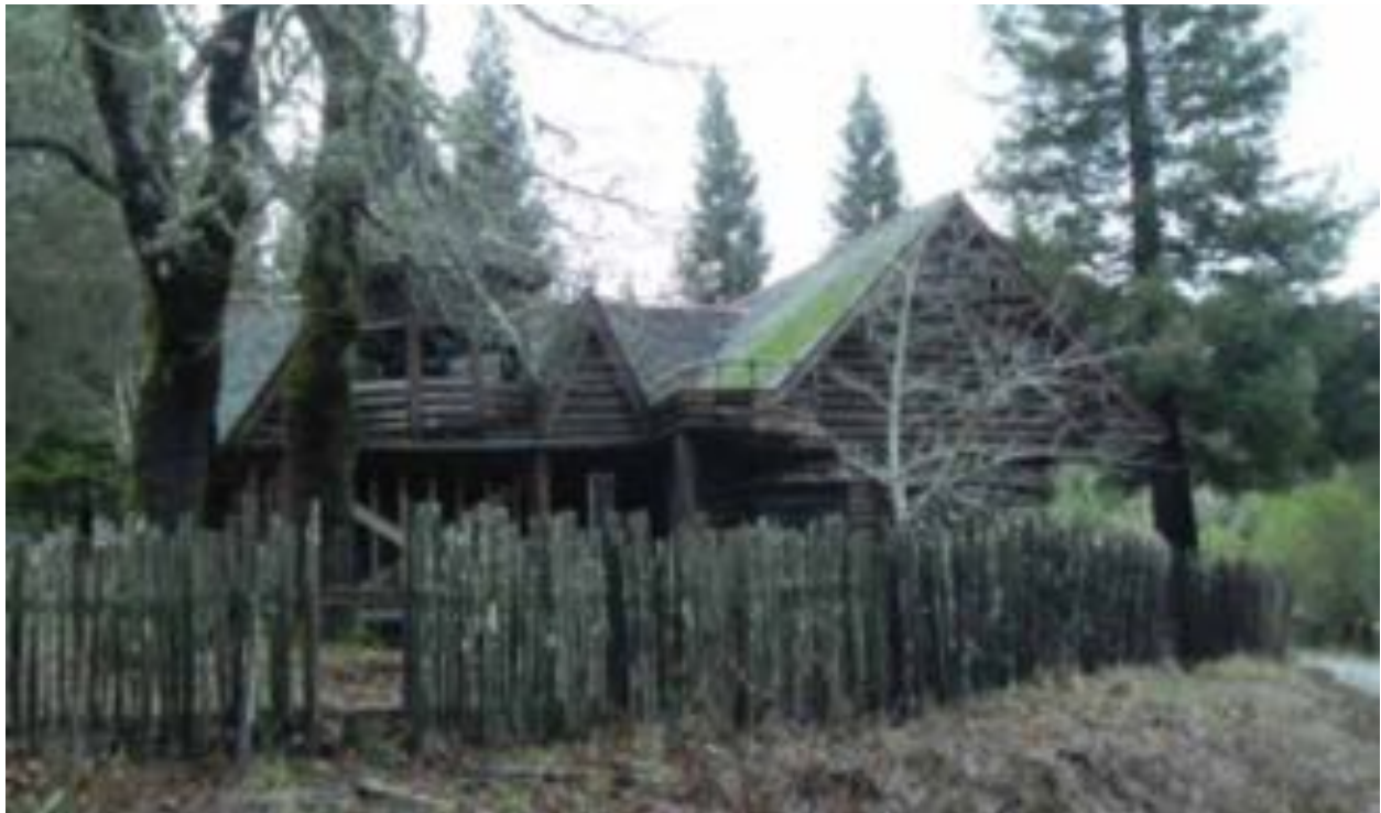
Fig.1 – PHOENIX CABIN - Front from fire road, looking north (MH-2014)
