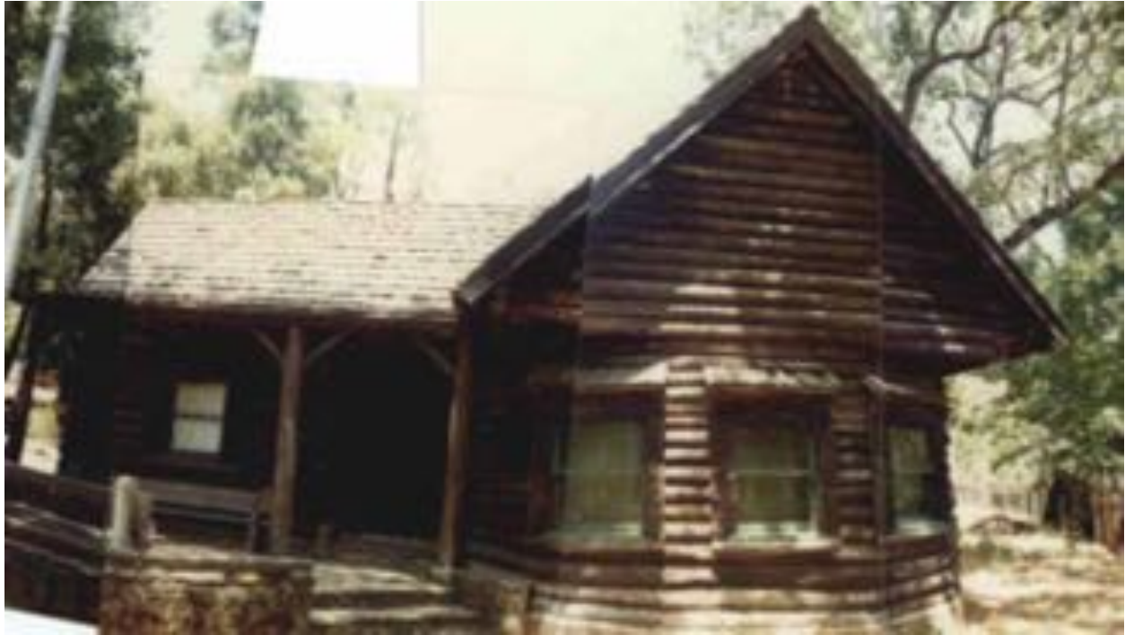
Fig.53 – Front, with previous porch - c1980s (MMWD)
