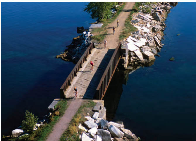
Raised trail with rip rap and bridge. Shown: Colchester Causeway, Colchester, VT.. Image credit: VT Fish and Wildlife Department
